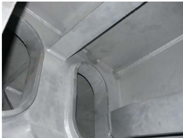
Day 14, after blasting with KinetiX: graded SSPC-SP10 near white metal finish
